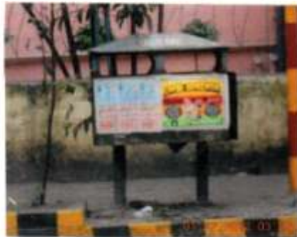
Kolkata Design Small & Wrong position of Inlet
